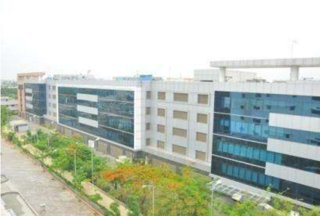
Figure-3 : M/s. TPCL, ELCOSEZ, Coimbatore
