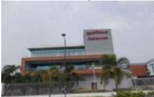
Figure-4 : M/s. Honeywell, ELCOSEZ Ilandhaikulam, Madurai
