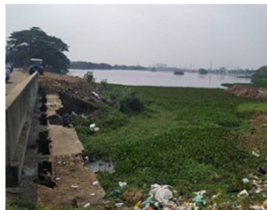
Outfall Sewer from STP at Chokkampungur
