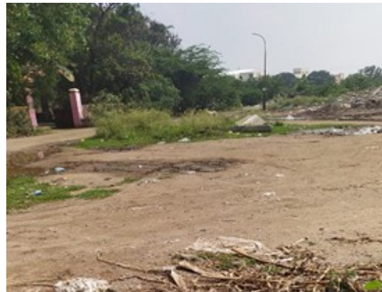
Sewage Treatment Plant at Chokkampungur
