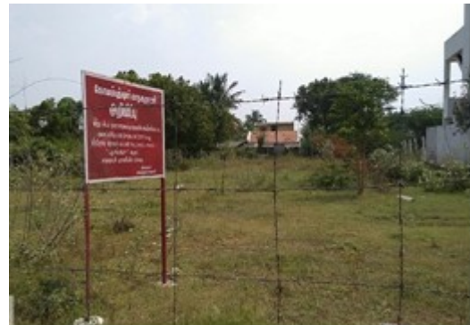
LIFT STATION-4 at Sri Ram Gardens
