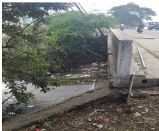
Outfall Sewer from STP at Chokkampungur
