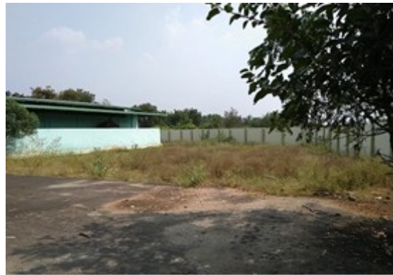
LIFT STATION-2 at Onapalayam Burial Ground
