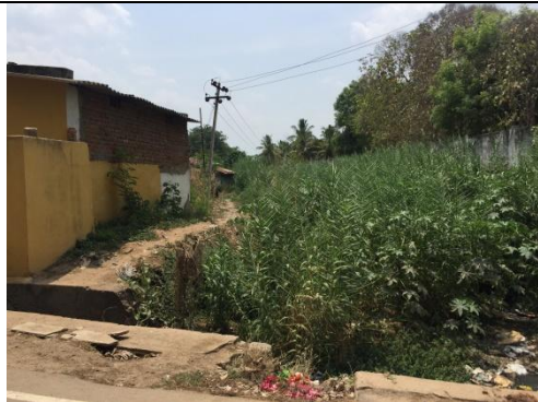
Pumping main alignment initially proposed within the drain alignment. However, considering social implications (houses close by and flooding during monsoon) alignment was changed in consultation with TNUIFSL, TWAD and ULB staff
